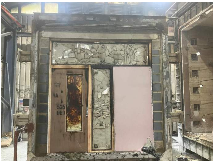
Figure 37 Unexposed face of the specimen at the end of the test
